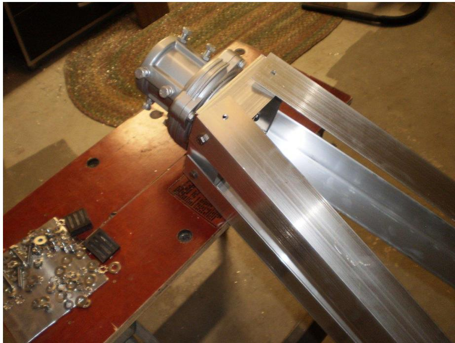
6. Tilt the assembled structure upright and spread the legs apart by about 32 inches (similar to unfolding a step ladder). Assemble the cross braces, upper shelf bracket (with rotor shelf mounting holes) and lower shelf bracket on each of the 2 open sides as shown below, using  $\frac{1}{4}$ "-20 x 1" bolts, lock-washers and nuts. Hand-tighten the hardware at this time.
